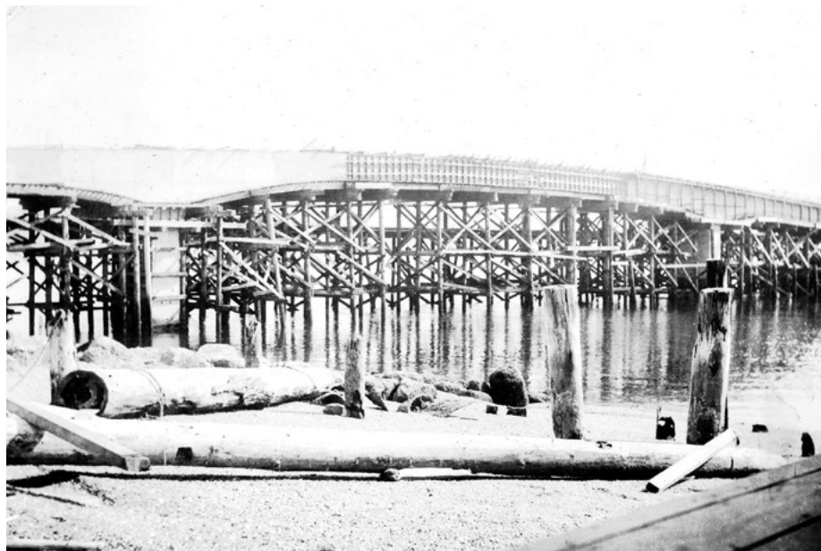
Support structure for the extensive formwork. Washington State Archives, WSDOT Records
