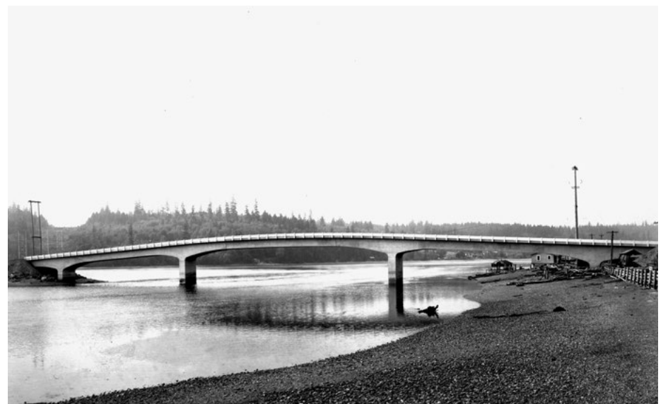
Photo by Asahel Curtis of the Purdy Bridge soon after it was completed in 1937. Washington State University Press
